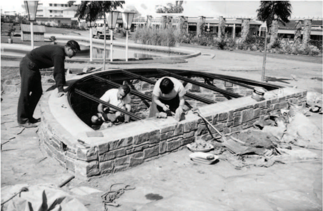
Figure 4: Museum staff building the showcase at one of the discovery areas, most probably the 1962 area. Photo: National Archives of Namibia
